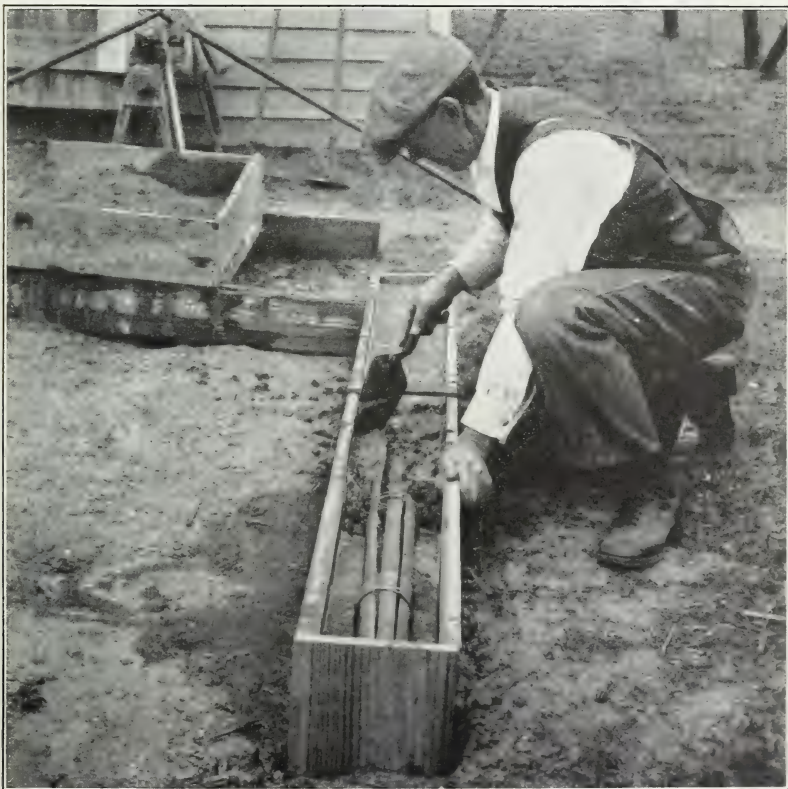
FIG. 2.—SPLIT BAMBOOS USED FOR REINFORCING CONCRETE POSTS
